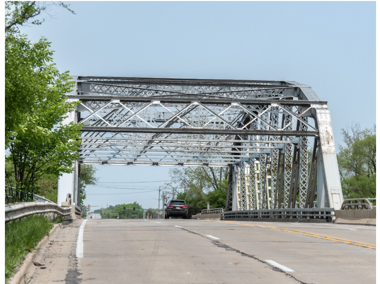
A car drives along the historic Cal Sag Channel Bridge.
